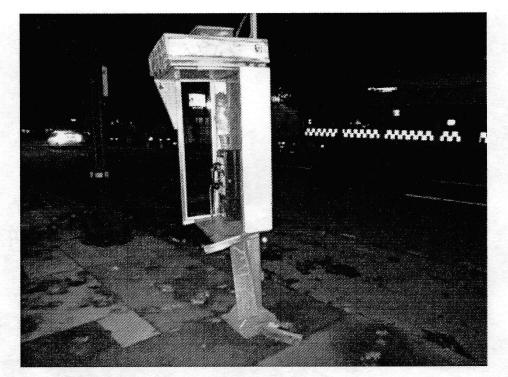
This phone kiosk was apparently hit by a car. A single bolt and cable stay kept it attached to the earth, but it seems like the enclosure and pedestal absorbed the impact, protecting the phone. It was gone a week later. Hopefully a collector picked it up and not a scrapper.
