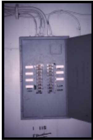
Fig. 2-9. Breaker panel.
