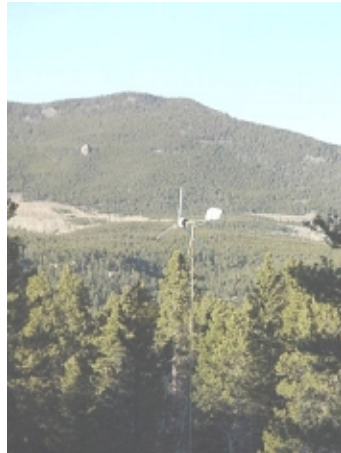
Homebrew turbines flying at pretty good sites, Colorado, USA. Both could use another 10-20 feet of tower (notice local tree heights)
