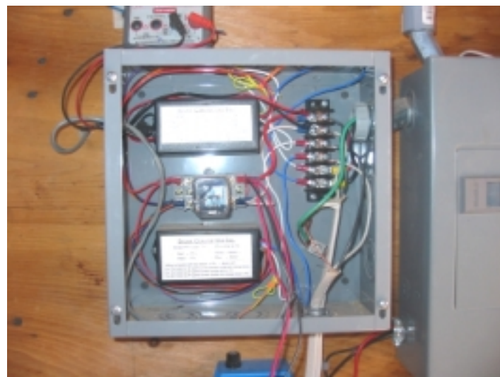
As you can see, the 10” x 10” junction box easily holds the two controllers, the bottle relay, and the terminal strips.
