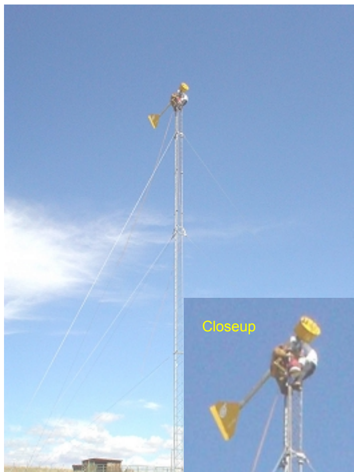
Professional wind turbine dealer, installer and mechanic Victor Creazzi of Aerofire Wind Power on a routine service call.
