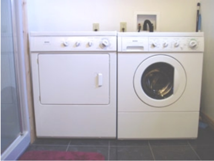
This Sears high efficiency clothes washer uses five-and-a-half times less energy than a similar sized unit. Coupled with the propane dryer to the left, this makes an excellent choice for any renewable energy based home.
