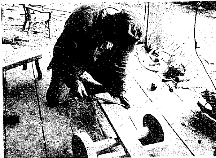
PLATE 278. The next step is to turn the wagon over, and shave off the sharp edges of the underside of the main support beam at the point where it will rest in the top of the front axle. This will allow it to turn on the front axle without binding.
