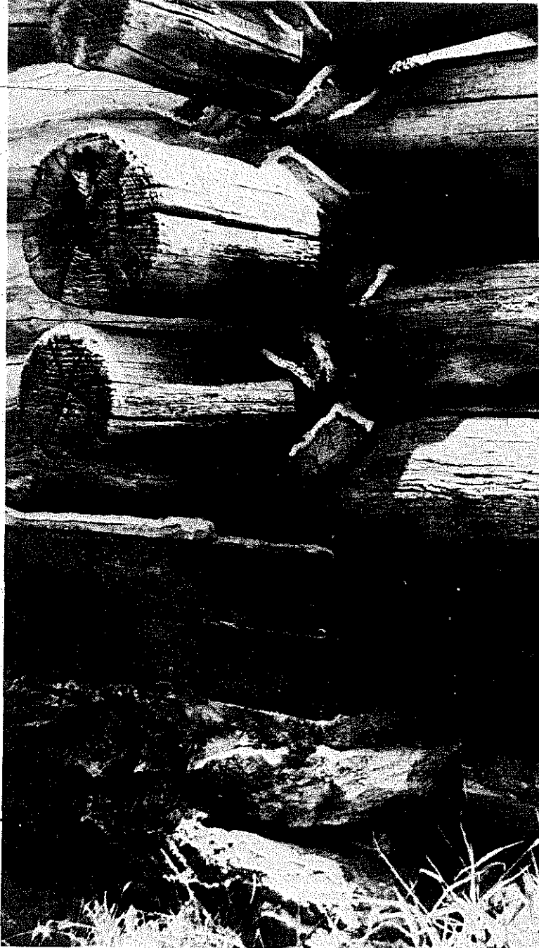
PLATE 60 The lap joint of this end log (arrows) fits snugly over the sill.
