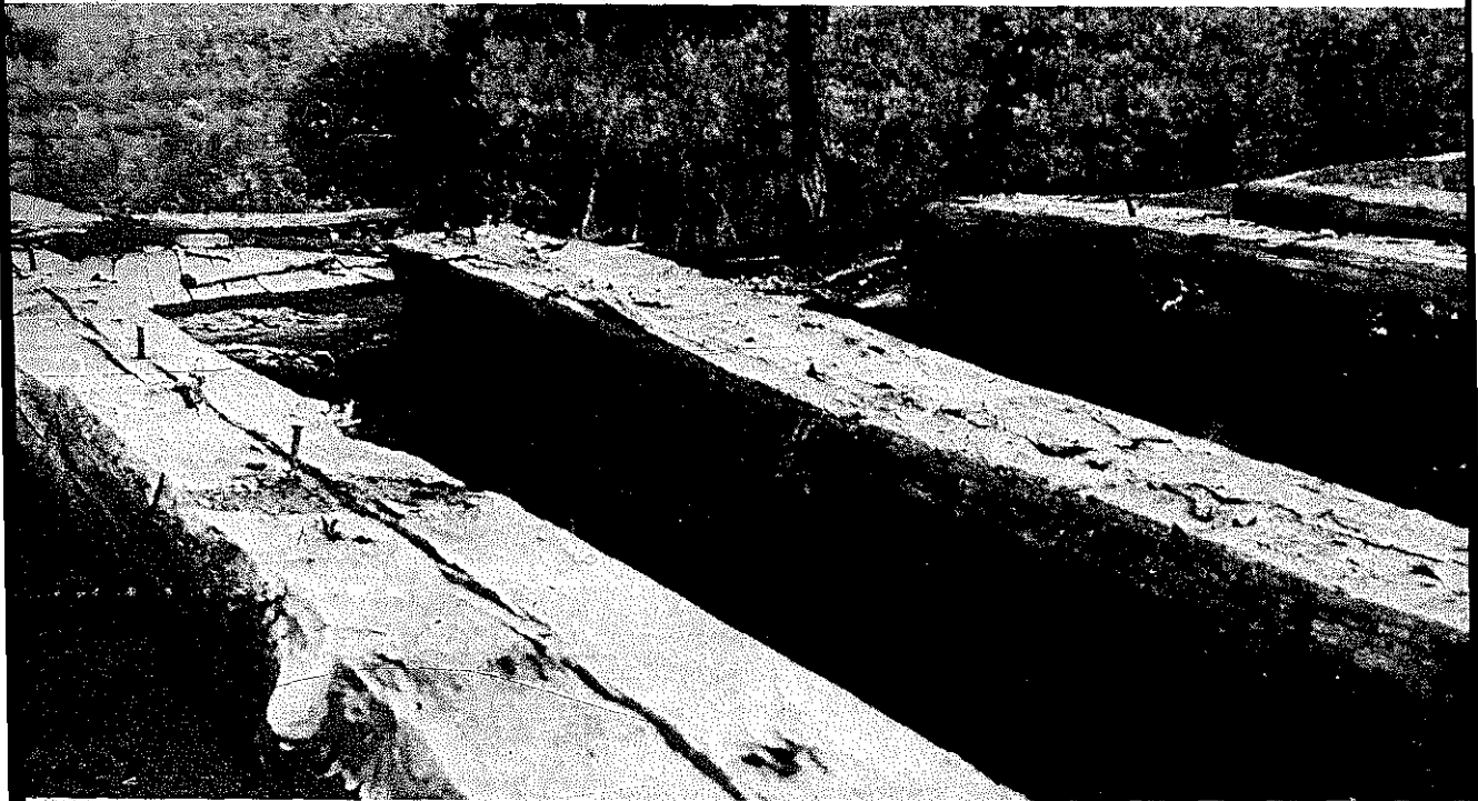
PLATE 56 These sleepers are lap-jointed at each end to fit the sills. A foot adze has been used to hew off their top surfaces. See also Plate 57.
