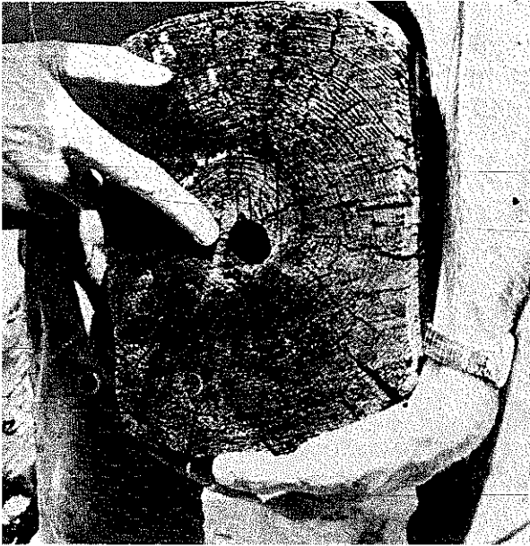
PLATE 133 A hole, drilled with an auger, into which the peg through the doorframe will fit.
