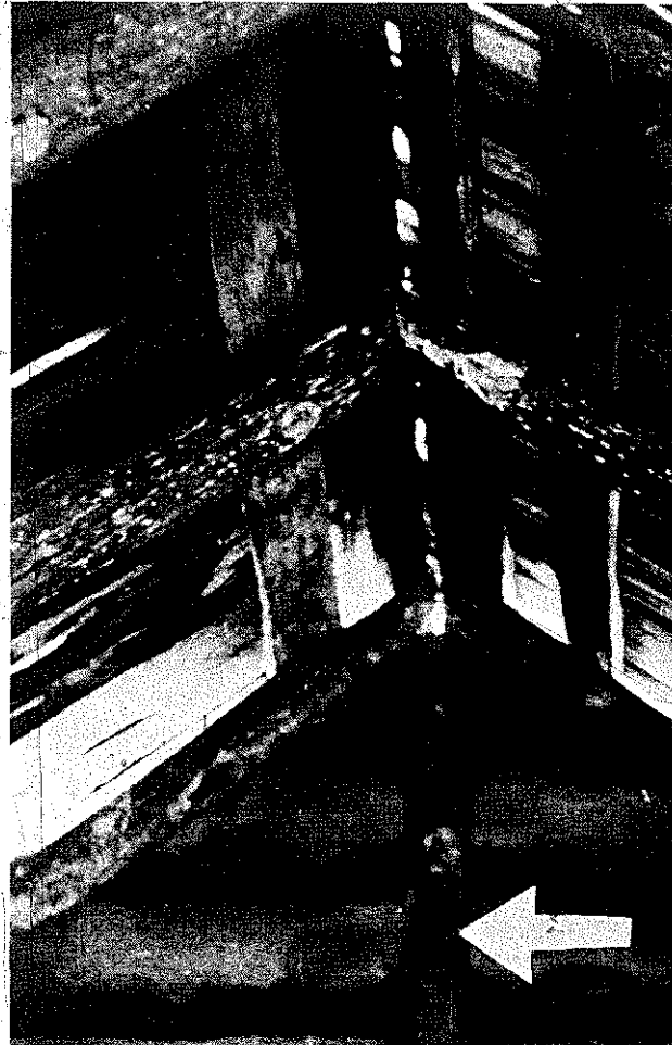
PLATE 121 From inside, center vertical support beam (arrow) for gable is visible. Note absence of ridgepole, and spacing of lathing for shingles.
