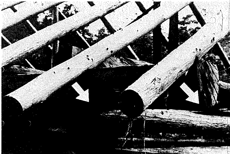
PLATE 101 Roy Thompson has extended his plates (between arrows) to support an overhang that will help protect the end of the cabin.
