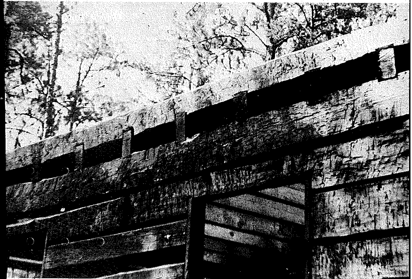
PLATE 100 In the South Carolina reconstruction, both the plate and the log above it are notched to fit the joists.
