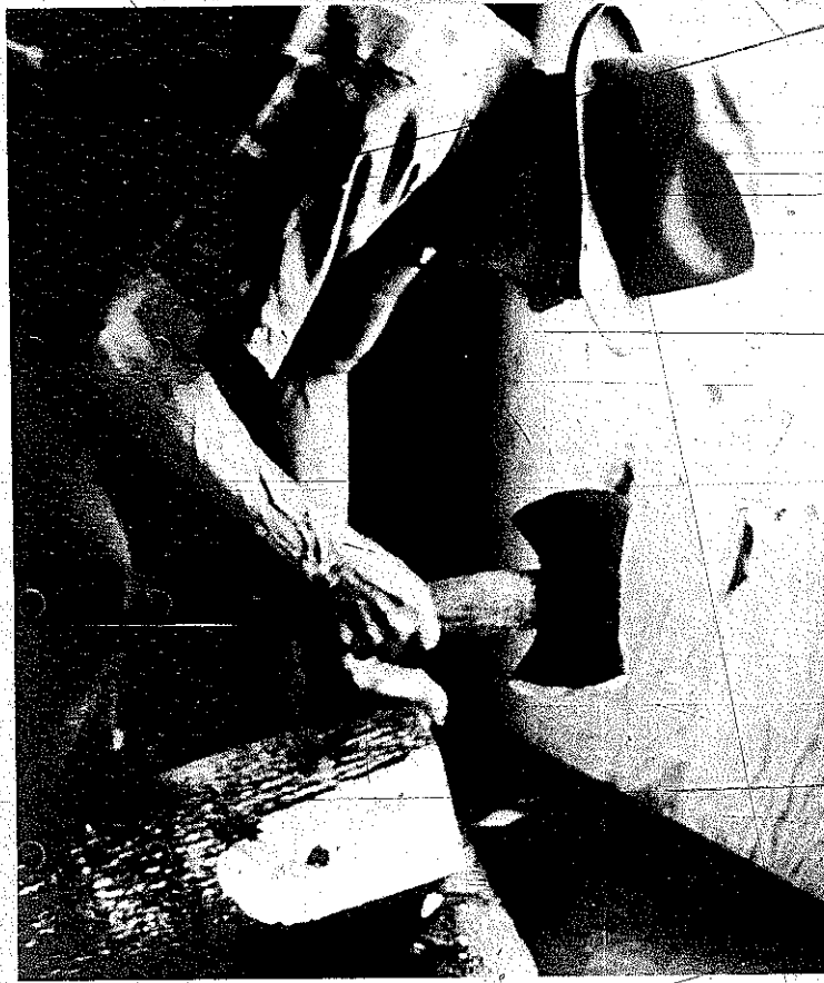
PLATE 62 With an axe, hew the two sides of the log back twelve inches from the end.
