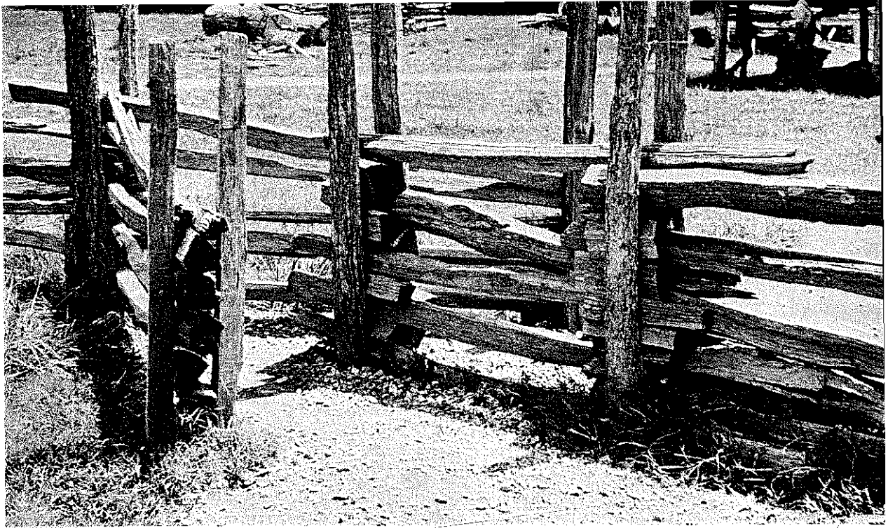
PLATE 6 A split rail fence in the reconstructed pioneer settlement at the Cherokee, North Carolina, entrance to the Smokies. The "V"-shaped opening eliminates the need for a gate that opens and shuts.
