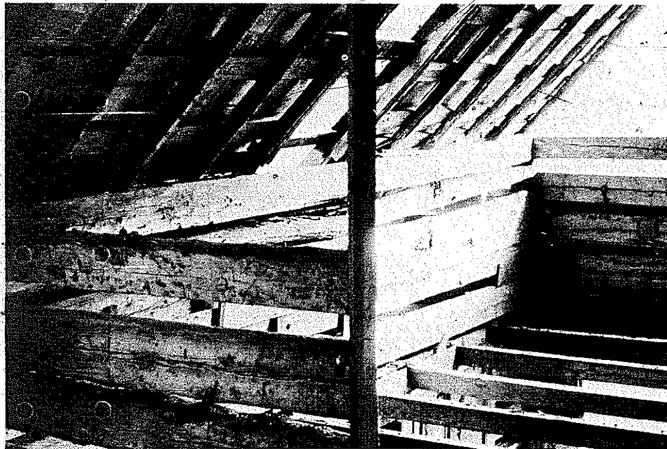
PLATE 94 The loft in this building rises five feet above the joists. Note the inside wall in the foreground.
