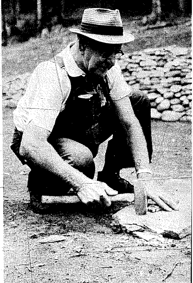
PLATE 149 Often the flagstones must be reshaped to fit. Claude measures the hole to be filled and then breaks the excess away with a hammer.
