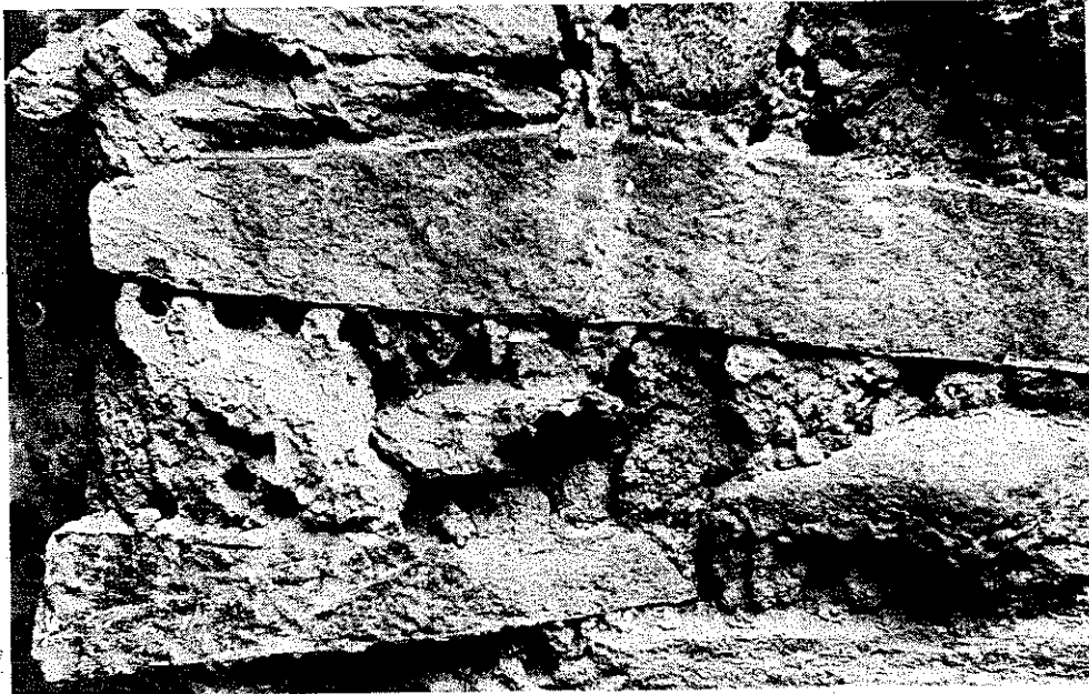
PLATE 144 A common problem with all-mud chinking was that it soon became the home for bees as the holes in this chinking show.
