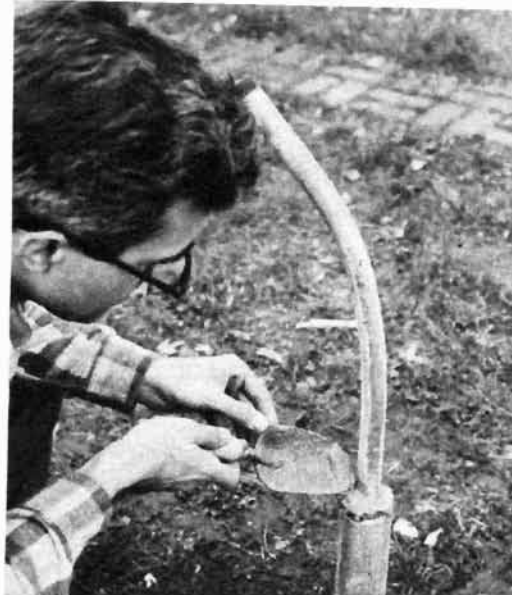
CEMENT the smaller pipe as shown so that it faces true North, not magnetic.
