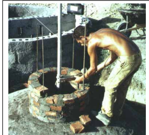
Figure 16: Construction of the digester neck with steel reinforcement Photo: Krämer (TBW)
