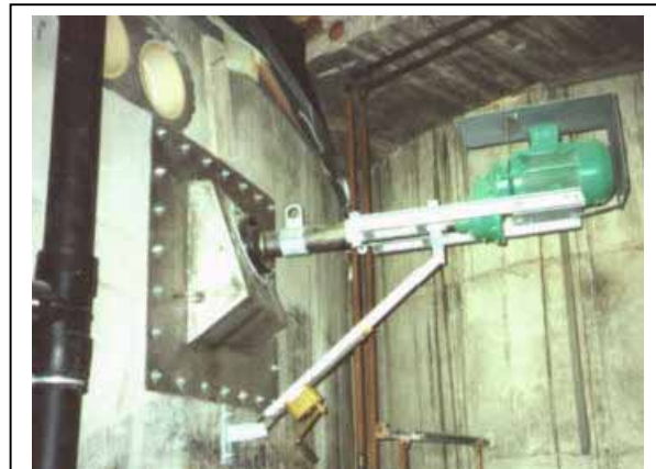
Figure 19: Stirring device for a european biodigester Photo: Krieg
