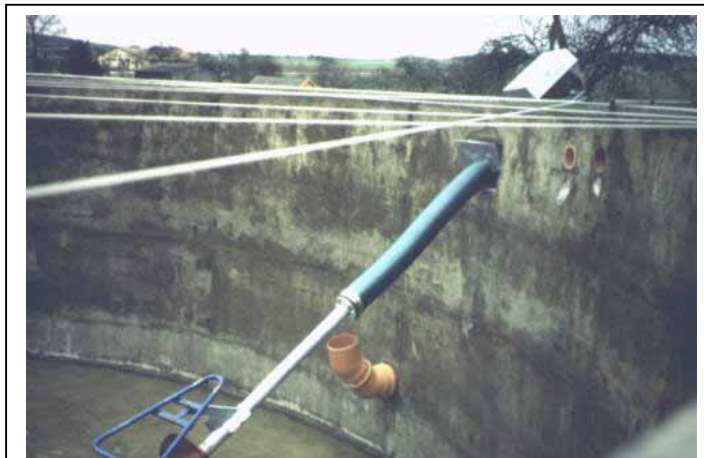
Figure 32: Mixing device in an agricultural digester under construction
