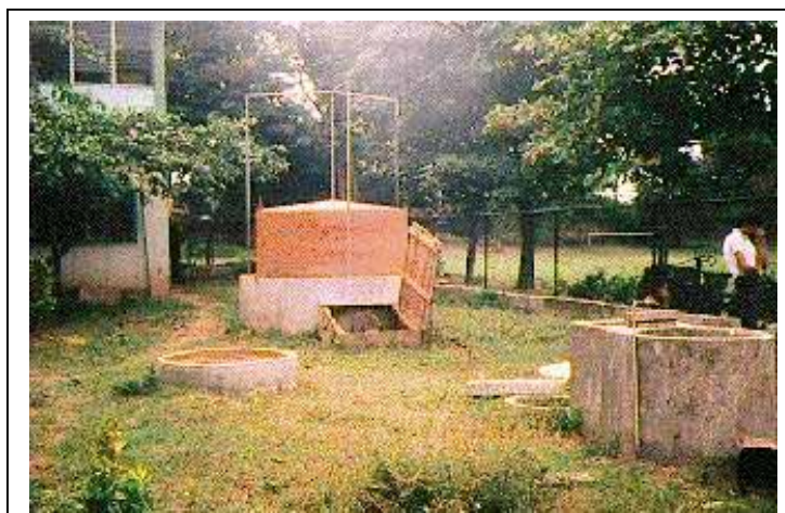
Figure 18: Biogas plant with separate gasholder in Nicaragua
