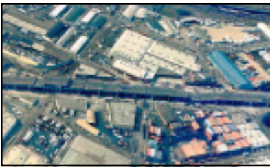
The collapsed section of the Nimitz Freeway.
