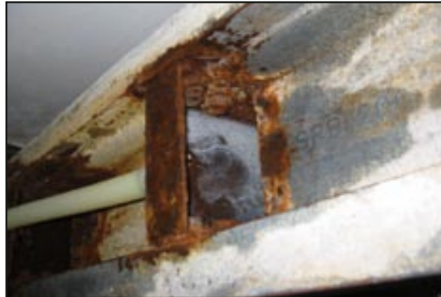
Examples of rust in the make and curing rooms.
