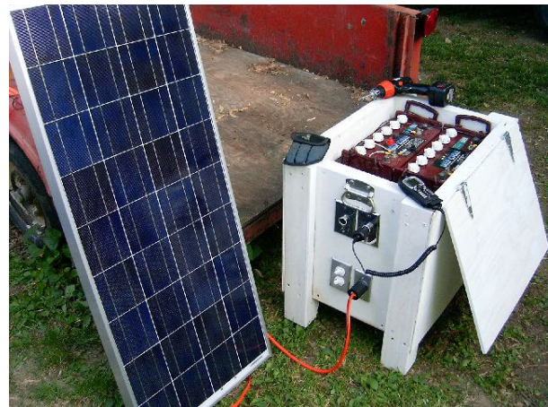
Connecting one of the solar panels for the first time.
